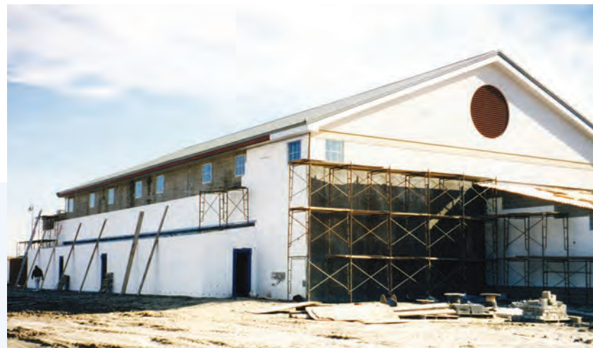
Community Center Under Construction Georgetown
