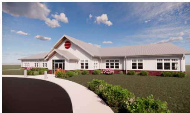
CHEER Administration & Support Services Building
